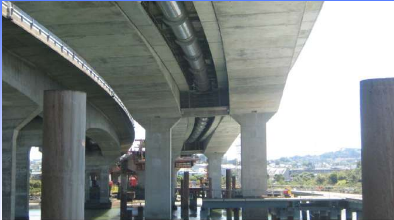
Pipeline suspension from span 4
