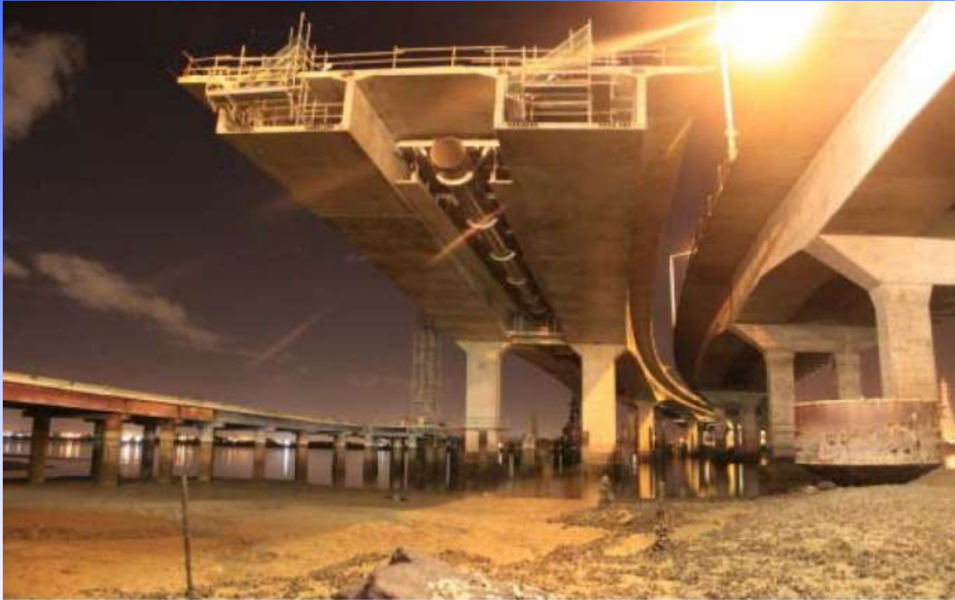
Suspended pipeline at the north end of Pier 5
