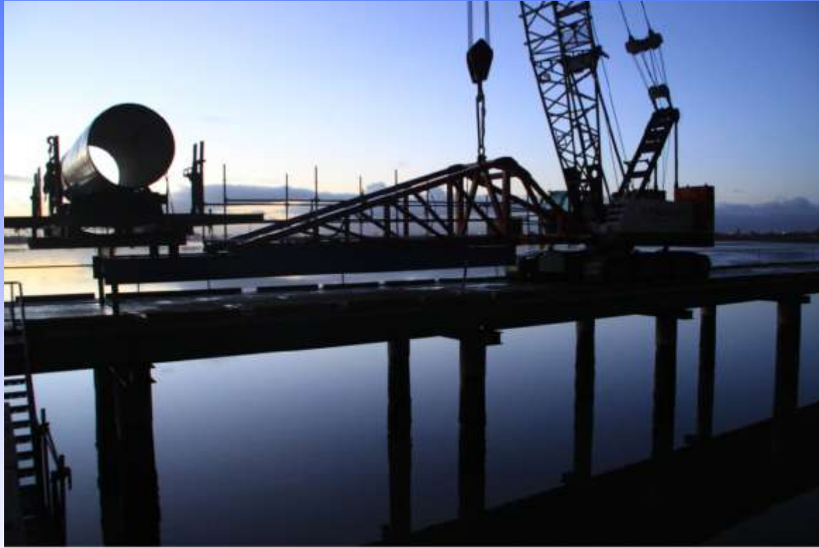
Suspended pipeline installation
